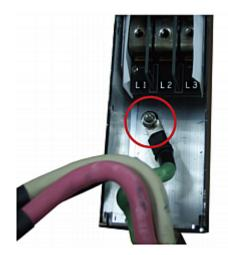
6. Fasten the ring terminals of all remaining wires to the terminal block and tighten each using a torque screwdriver. The appropriate torque settings vary according to the screw size.
